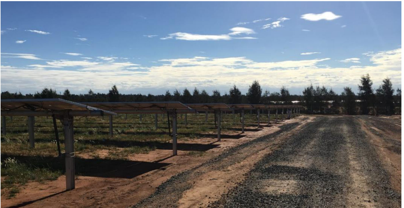
Internal Roads Completion
